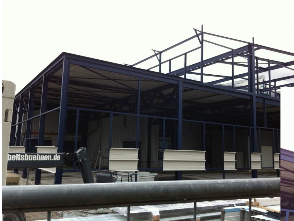
North-west corner October 12, 2011
